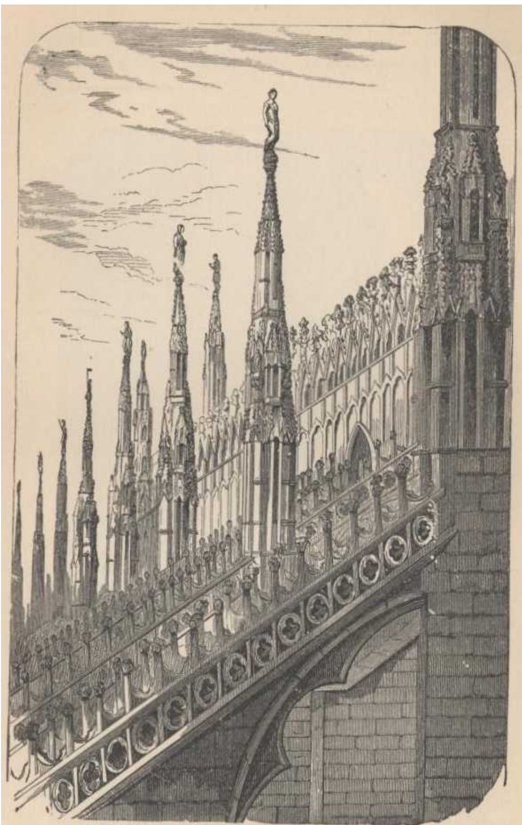
ROOFS AND SPIRES OF CATHEDRAL AT MILAN.
